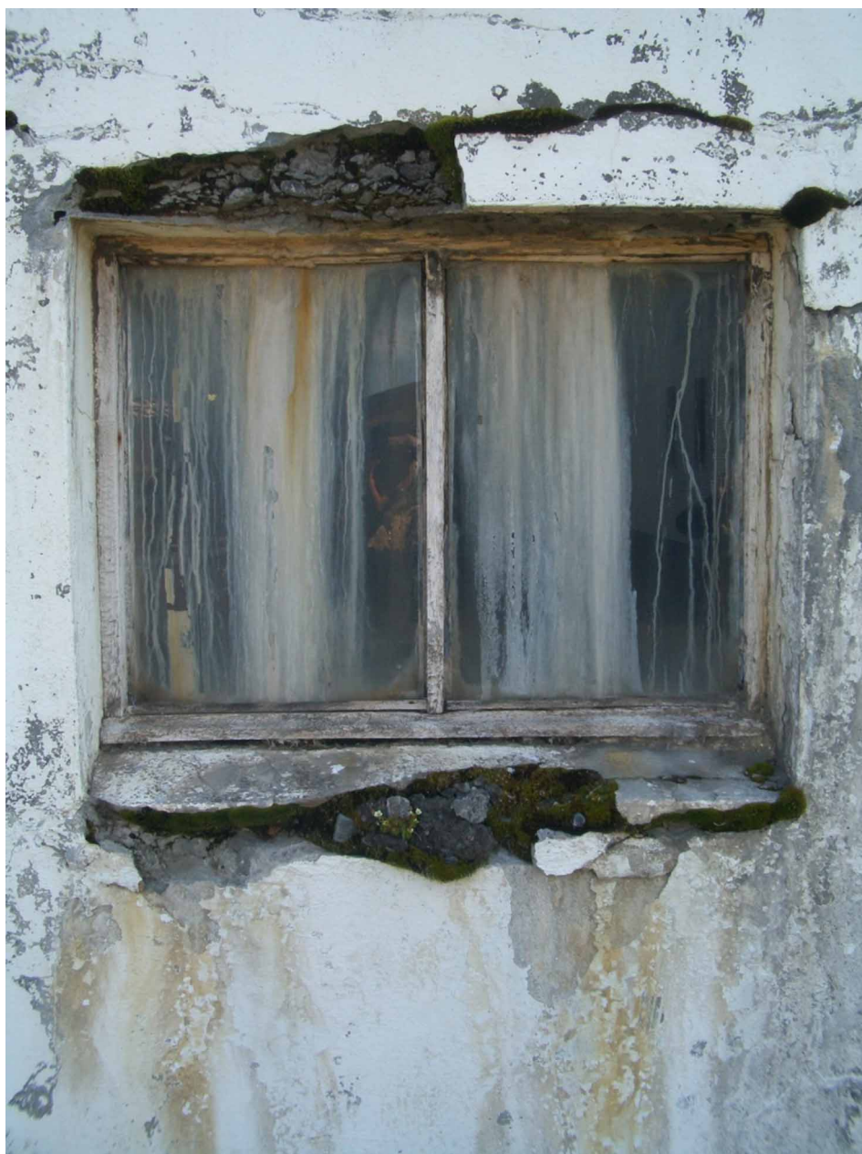
Figure 4. A window of the factory where moss and grass is growing through the cement. Image: Gunnar Thór Jóhannesson.
